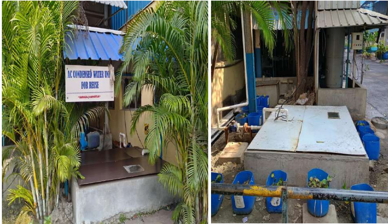
Photo: A/C condensed water reuse stations.
